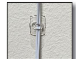
Alternating each clip's openings left and right helps keep the wire in place as it runs up the wall. Keep the openings facing up when running horizontally.
